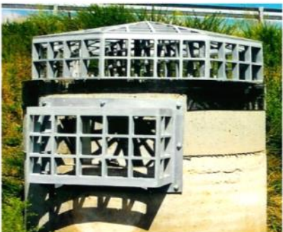
Dulles Toll Road, VA
