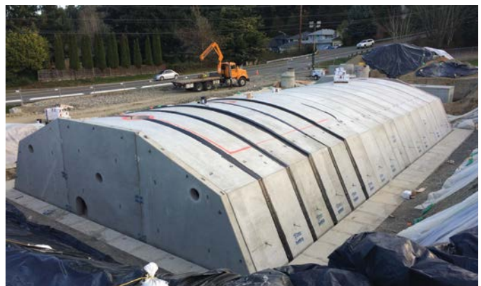
CON/SPAN® O-Series® Detention utilizes EXPRESS® Foundations for faster installation.
