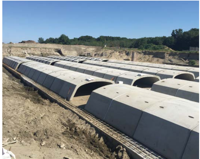
CON/SPAN® O-Series® Detention utilizes EXPRESS® Foundations for faster installation.
