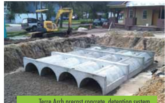
Terre Arch precast concrete detention system
