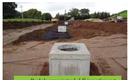
Manhole access instead of 4" inspection port
