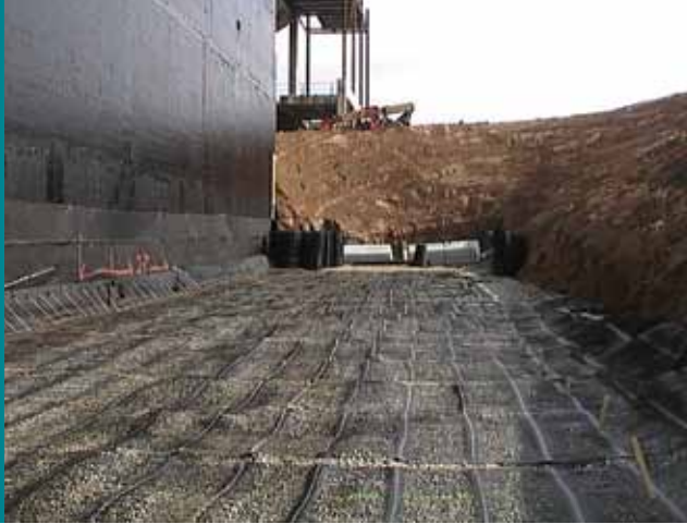
The John Paul Jones Arena at the University of Virginia combined the Geopier System in lieu of drilled shaft foundations, with a SierraScape® Pressure Relief Wall to eliminate costly concrete foundation walls.
